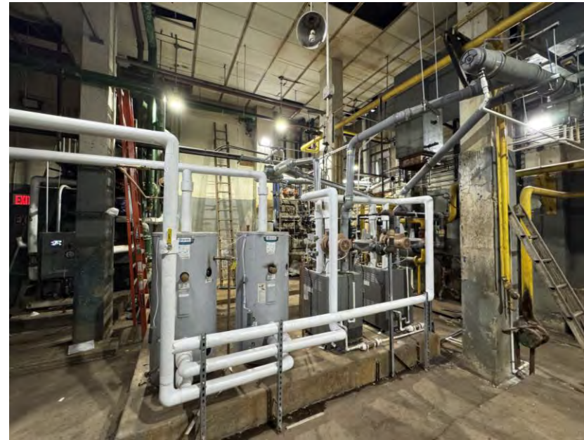
Volume Water Heaters and Storage Tanks
