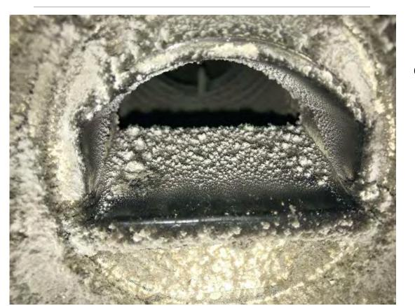
A four year old 20 story building located in Long Island City, with clogged CAR dampers unable to modulate.
