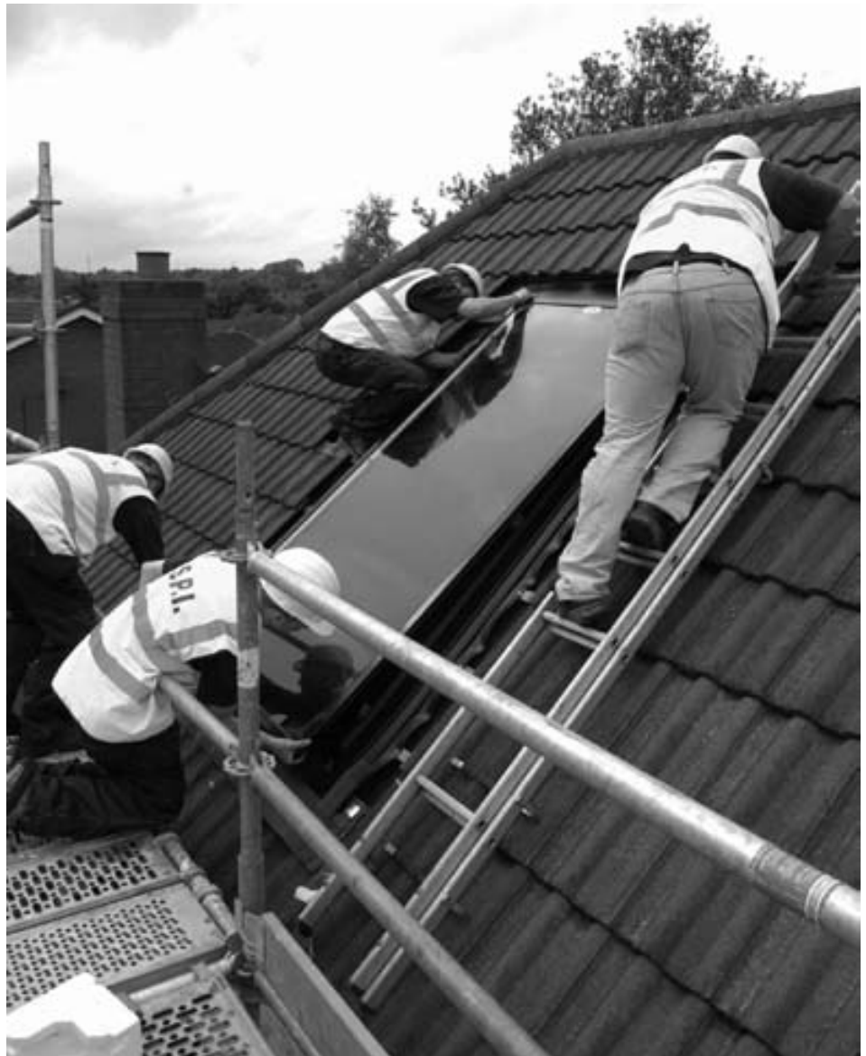
A team of professional solar installers
