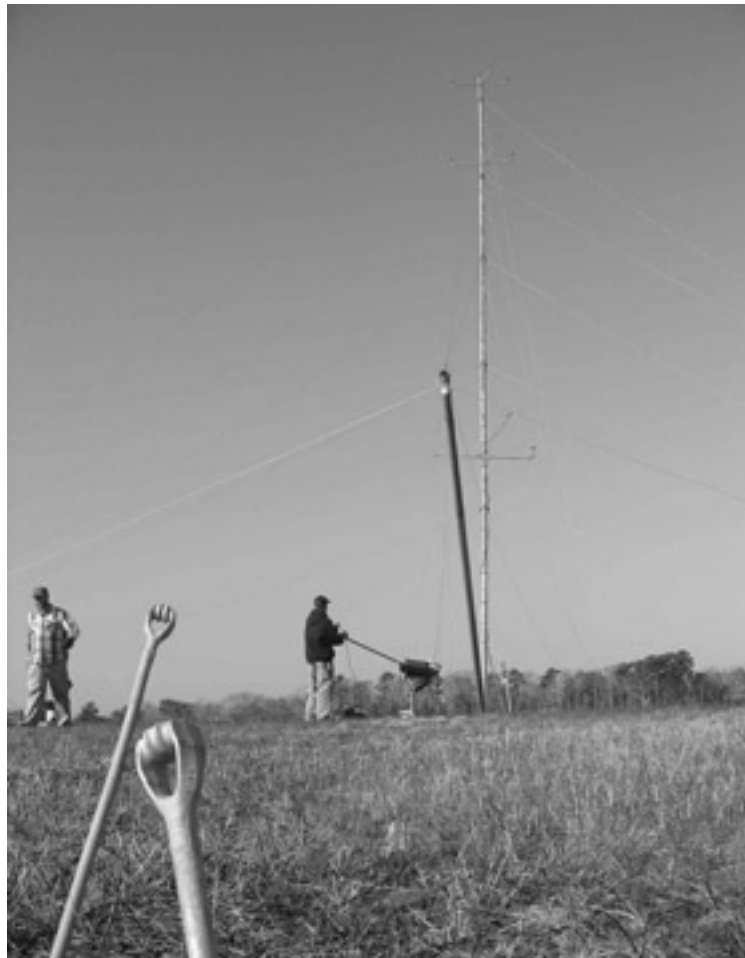
A meteorological tower goes up in Falmouth, MA. This tower was erected in April 2004 and is currently collecting wind data for the site.
