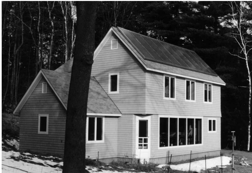
This superinsulated house in Hanover, NH uses the equivalent of 55 gallons of fuel oil annually for heating and hot water.
