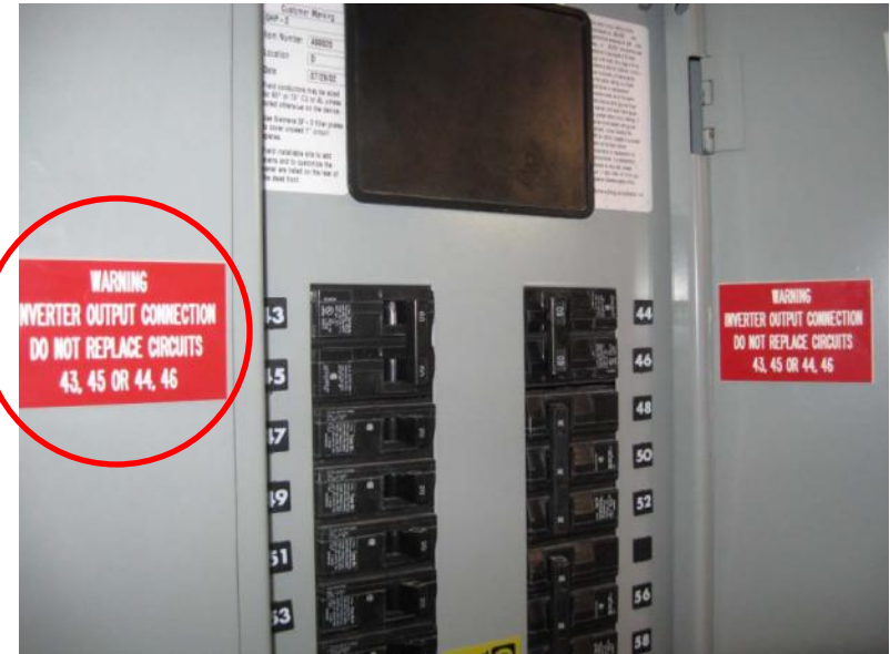
ABOVE: Photo of bus bar showing two relocated 60-amp breakers and appropriate labeling.
