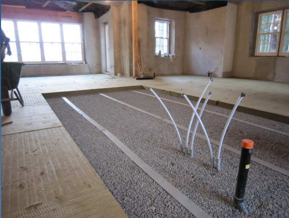
Toprock installation in British Columbia - Photo: Roxul
