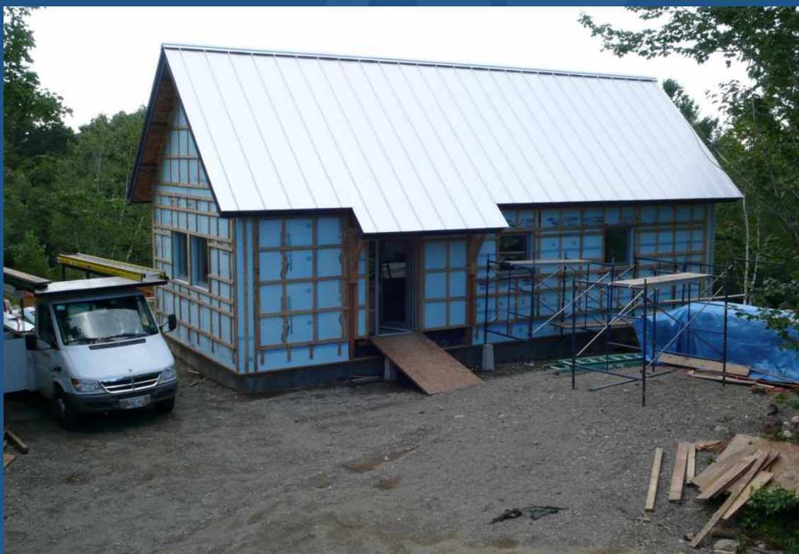
Net-zero-energy house with 4" XPS wrapped around 2x6 walls with cellulose. Photo: Bensonwood
