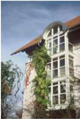
Shafbruhl Housing, Tubingen, Germany. Stucco terra cotta exterior mass walls with wood beams and terra cotta planks. Architect: Joachim Eble
