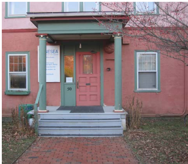
Non-accessible main entrance
