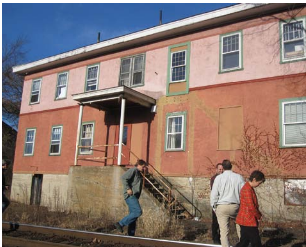
South elevation along railroad tracks - showing stucco at the end of it's useful life
