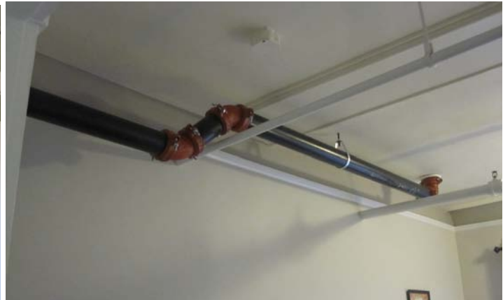
Existing sprinkler system
