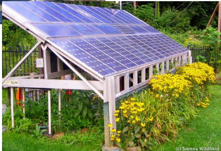
The existing 3 kW park PV system
