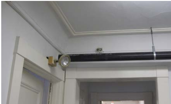
Existing historic trim is visible along most of the second floor walls and on the doorways.
