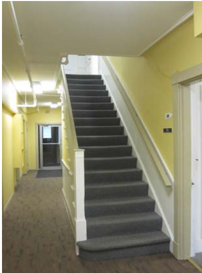
Historic central stair
