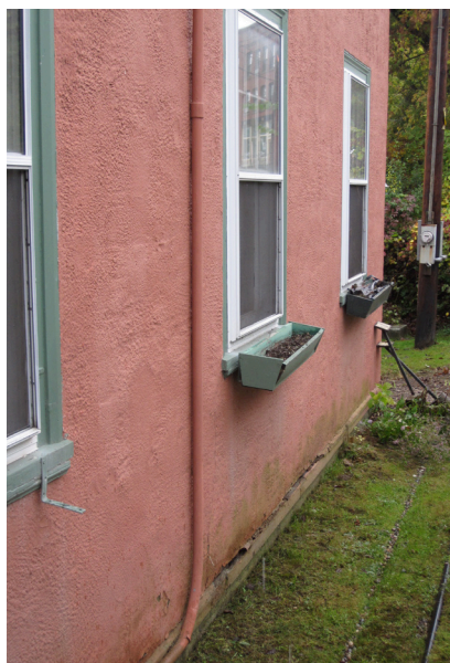
Deterioration of the stucco at the base of wall
