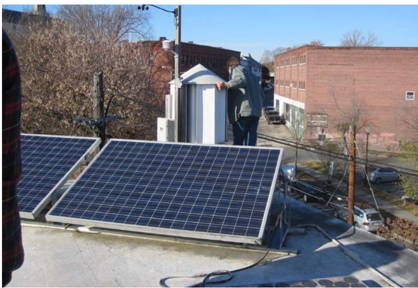
Roof with 1.5 kW photovoltaic system.
