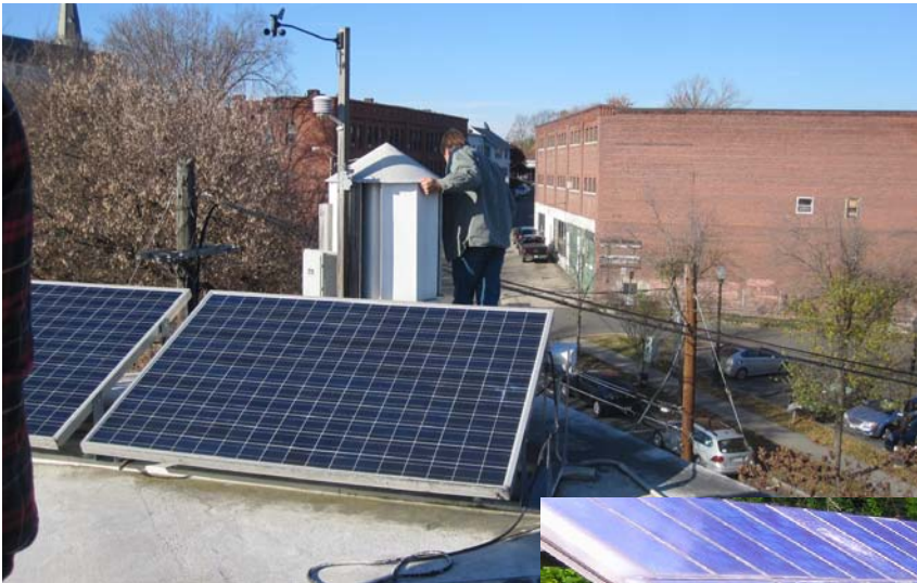
The existing 1.5 kW roof top PV
