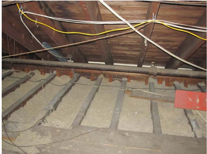
Attic cellulose insulation
