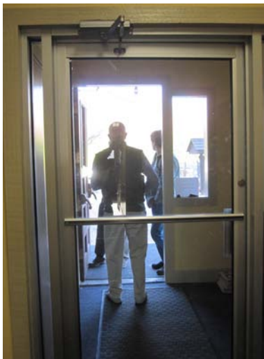
Code-acceptable entry vestibule
