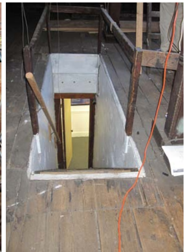
Attic access stairs
