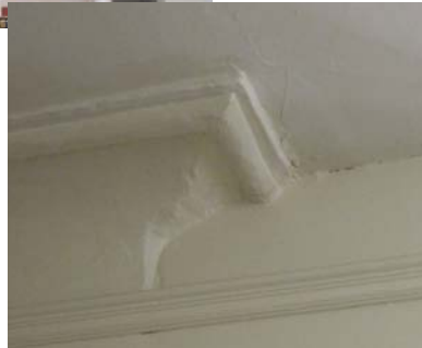
Existing historic trim is visible along most of the second floor walls.
