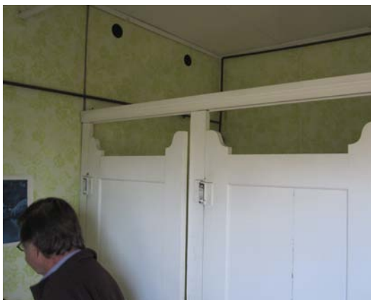
Non-accessible bathroom stalls
