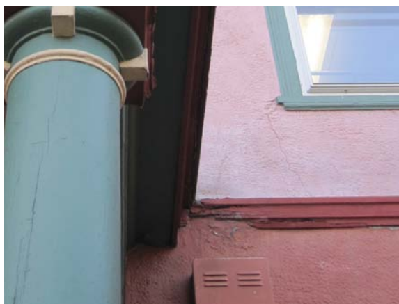
Deterioration of horizontal wood trim
