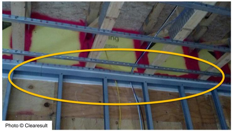
Determine the optimal air barrier plane
