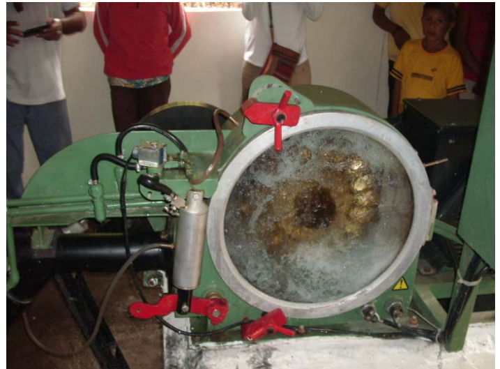
Photo 2. Examining the Pelton wheel generator.
